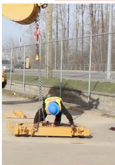
Move rigging to the top of the strut and place in strut stands.
