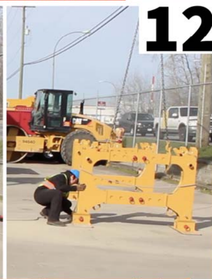
Move rigging to the top of the strut and place in strut stands.
