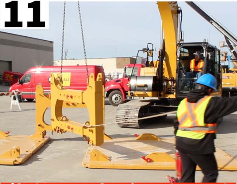
Lift the struts free from the panels
